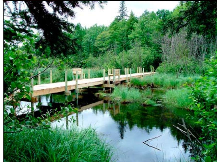
A view of the Plumbago Creek Valley during the peak of autumn color (upper photo), and a close-up of the six-foot-wide, 156-foot-long span over a wetland and beaver pond area of the creek. Approximately 2000 volunteer hours and a few thousand dollars went into this project -- not including in-kind materials from lumber harvested and milled nearby. (Photos by Doug Welker)
