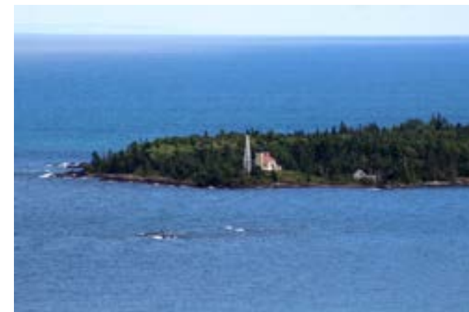
Copper Harbor Lighthouse by Brian Doyle
