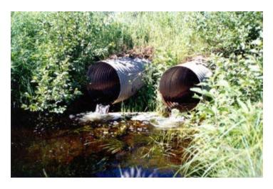
The worst possible stream crossing is a "perched" culvert (above.) Fish would have to jump to enter the downstream end of this culvert and then make its way with high velocity over the steel corrugation which is normally impossible. There are numerous examples of perched culverts around the Western UP where I managed trout for the DNR during my career. Many other culverts are undersized and block trout with flow velocity or placement that is too much for trout to swim upstream through them.
